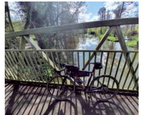
Byfleet, bridge over the River Wey
